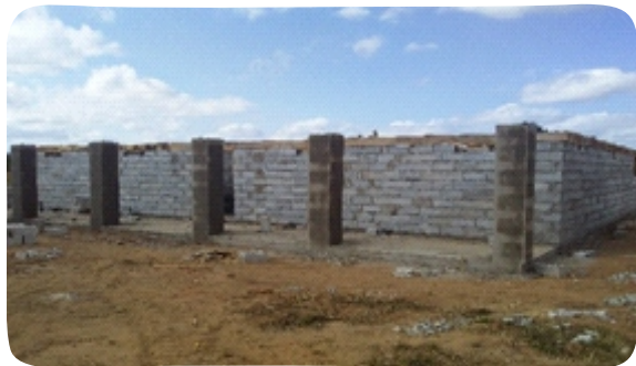
Rufunsa Community Seed Bank under construction
